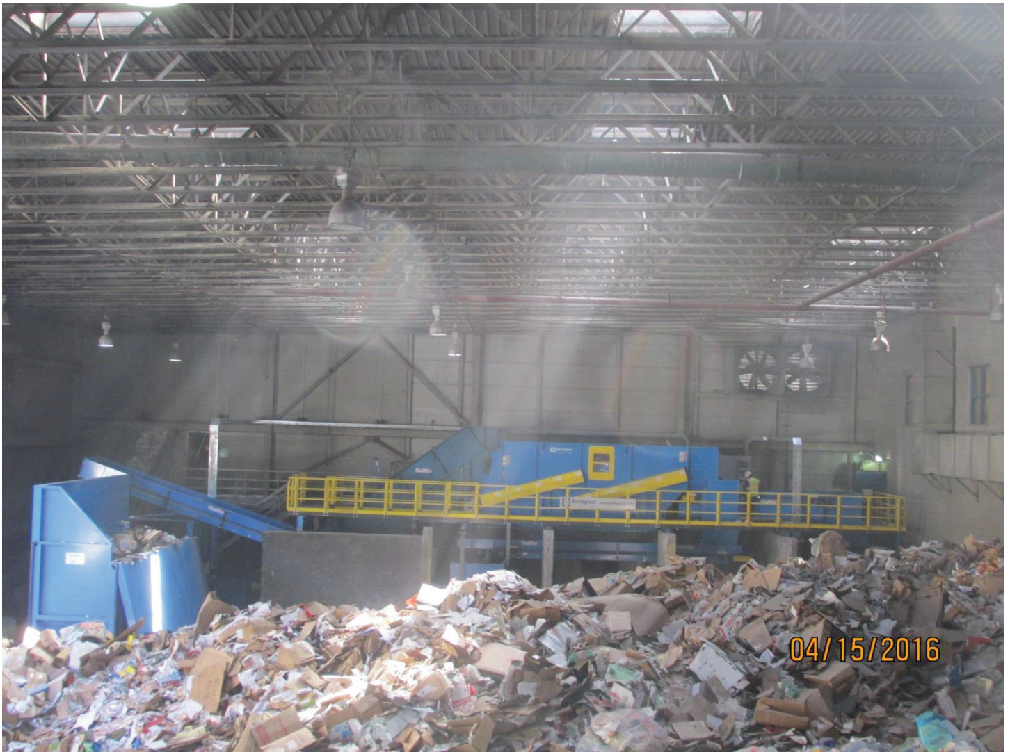
Mixed paper and cardboard at the Material Recycling Facility (MRF) in Yonkers.
